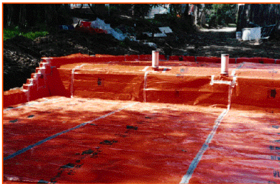
Kordon TMB Full Under-slab showing flexibility with stepdowns
