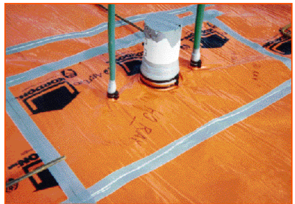
Multiple Penetration - Kordon TMB - full underslab
