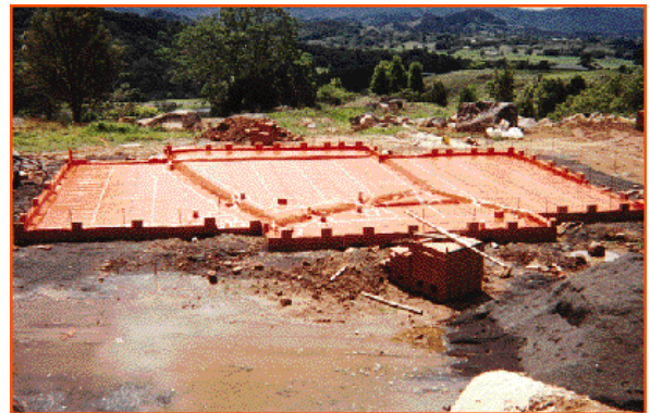
Kordon TMB Full Under-slab
