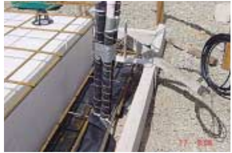
photo 2 showing multiple pipes each protected with Kordon
