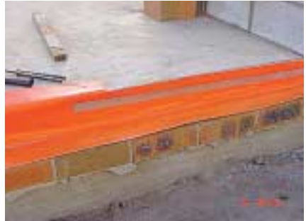
if tiling is to extend to slab edge Kordon TB is installed as shown - secured with gal hoop-iron/strapping.
